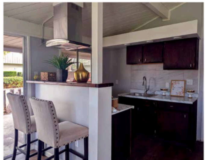
Renovation of one of the units. Photos by Doreen Gounard.
